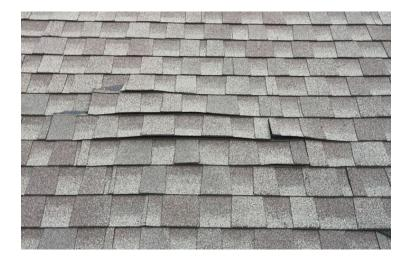
This bulge is due to the decking being misshapen by moisture and heat over time due to poor ventilation. Windstorms have lifted and damages the shingles further.
